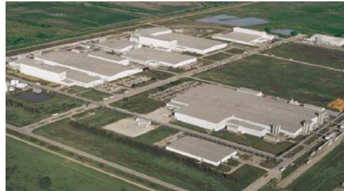
Our 700-acre Plant in Lolita, Texas
